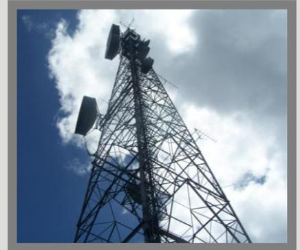
Tower infrastructure required for solid parabolic antennas
