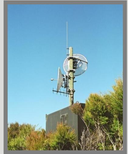
Typical lightweight grid style parabolic antenna
